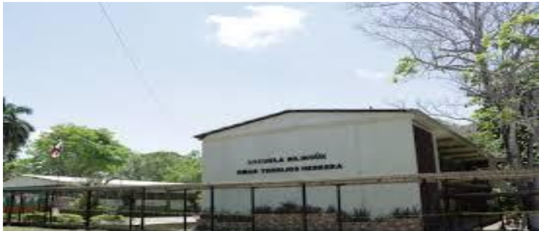
Photo 2. Structure of the Omar Torrijos Herrera school.
